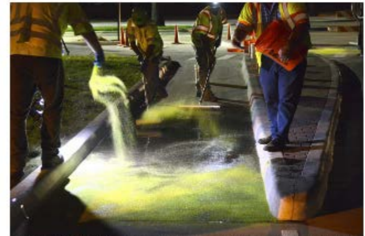
Researchers at Texas A&M University say they have designed an innovative bike lane that incorporates futuristic design with glowing paint. They also installed it on campus. (Texas A&M)
