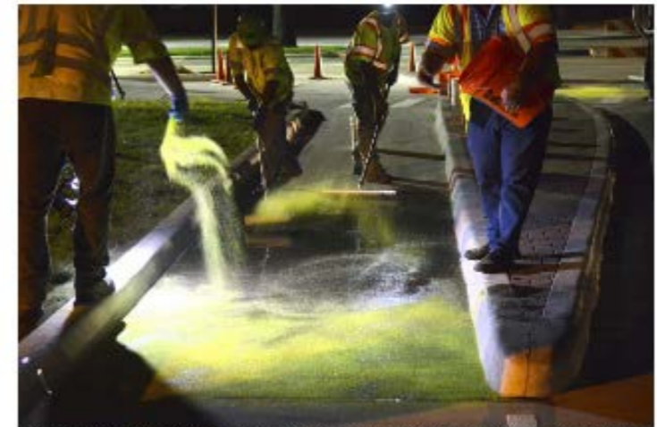
Researchers at Texas A&M University say they have designed an innovative bike lane that incorporates fluorescent paint with glowing mineral. They also installed it on campus. (Texas A&M)
